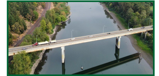
60-year-old West Camas Slough Bridge
